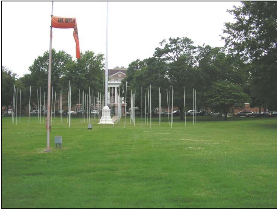
Photo 2-4a – View looking north to Building 1 at Flagpole
