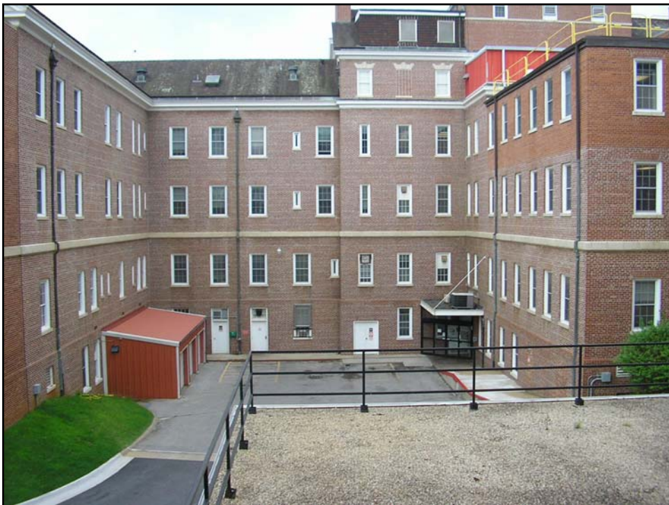
Photo 2-4f – Location of Pharmacy Addition. Rear of Building 1.
