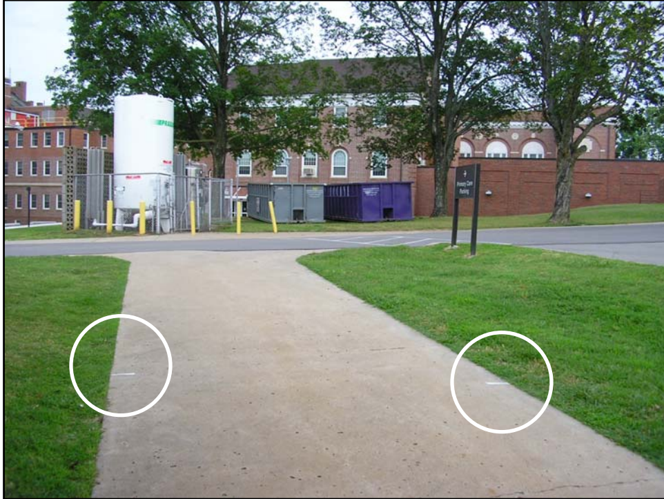
Photo 2-4g – View from walkway at Building 37. (Circled white paint marks indicate location of addition exterior wall)
