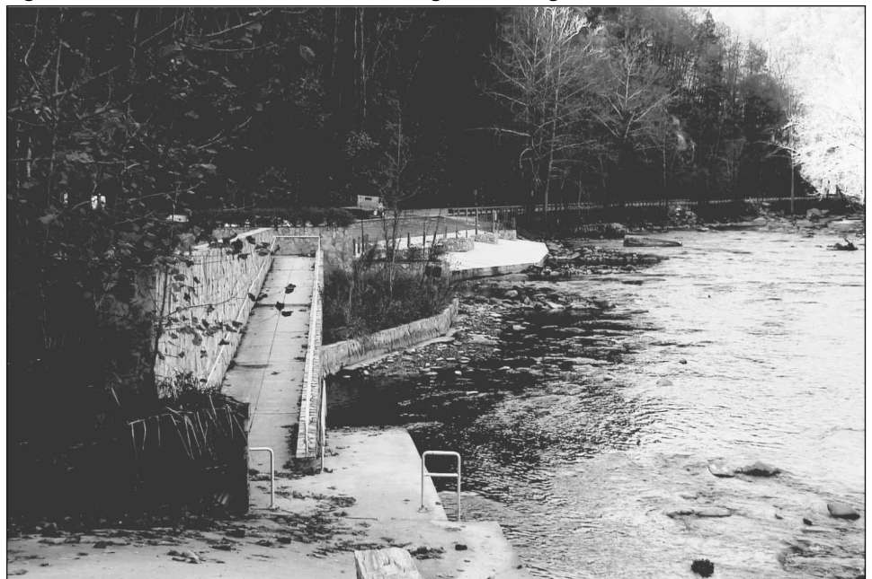
Figure 2: Enhancement of Boat Launching Area along the Nantahala River
