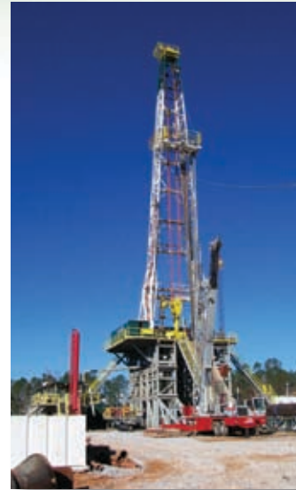
Well drilling rig
