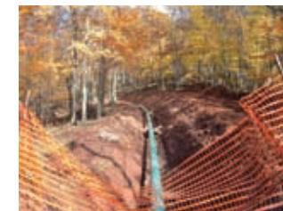
Pipeline in trench
