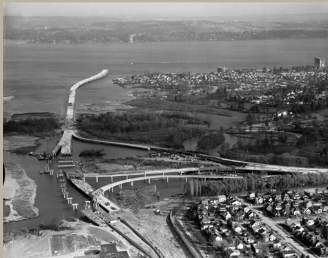
Aerial view of Evergreen Point bridge under construction in 1963
