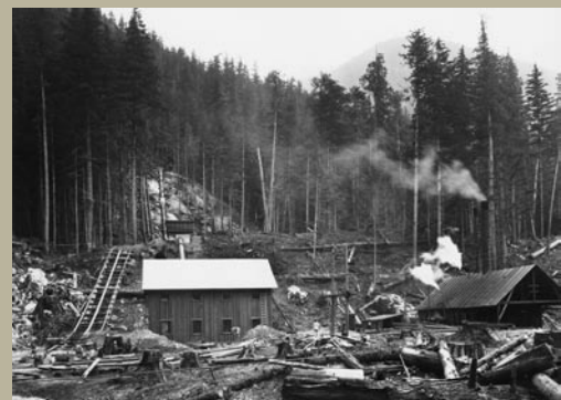
Skagit Dam construction site, 1921
