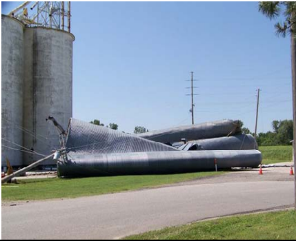
A bow echo raced across south-central and southeast Kansas during the evening hours of June 3 rd , 2008, producing numerous reports of 60-80 mph wind gusts. The severe winds toppled trees, downed power poles and caused some structure damage. Pictured above are two destroyed 80,000 bushel grain bins near Winfield. Photo courtesy of Brian Stone.
