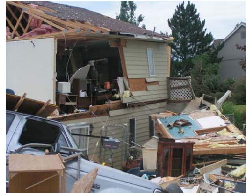
EF3 tornado damage from the June 11 th tornado just southeast of Salina. The damage shown above occurred near the intersection of East Schilling Road and South Holmes Road. Wide-spread damage was noted to several homes, businesses, and trees along the tornadoes 16-mile path. Total property damage was estimated at roughly 2.63 million dollars. Amazingly, no injuries were reported. The same storm system went on to produce the strong and deadly Chapman and Manhattan tornadoes.
