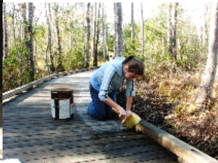
Applying sealant to boardwalk
