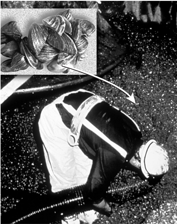
Worker standing inside a water intake pipe removing zebra mussels
