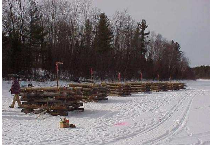
A series of fish cribs are placed on the ice along a lake's shoreline on the Washburn district.
