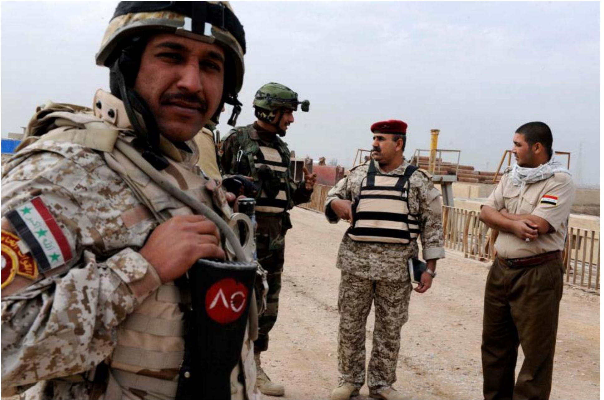
Iraqi soldiers gather around in order to assess and discuss repairs to the water pump filtration system on a dam, on Jan. 1, 2009 in Basra, Iraq.
