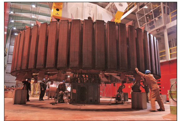
Niagara project generator undergoes overhaul.
