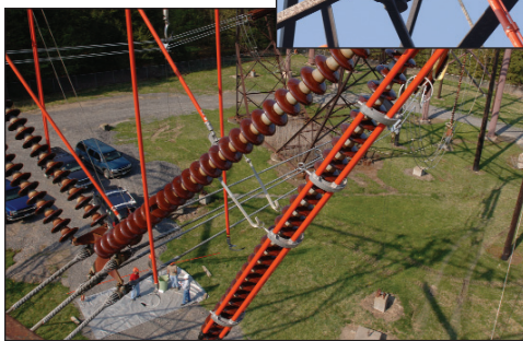
Top: Maintenance crews lower transmission line insulators to replace damaged disks. Center left: Steve Palencar demonstrates use of hot stick. Center right: Tom Bartolomie, left, directs apprentices Gregg Baker, middle, and Todd Jones. Left: Bird's-eye view of insulators and hot sticks.
