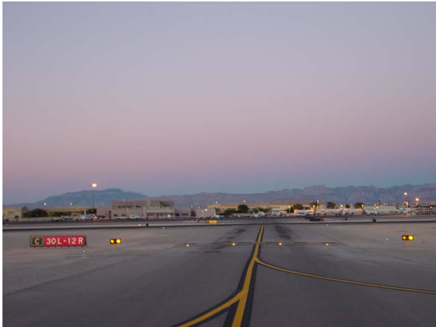
Figure A-2. Delta 2—Runway 12R-30L and Taxiway C (Northeast side)
