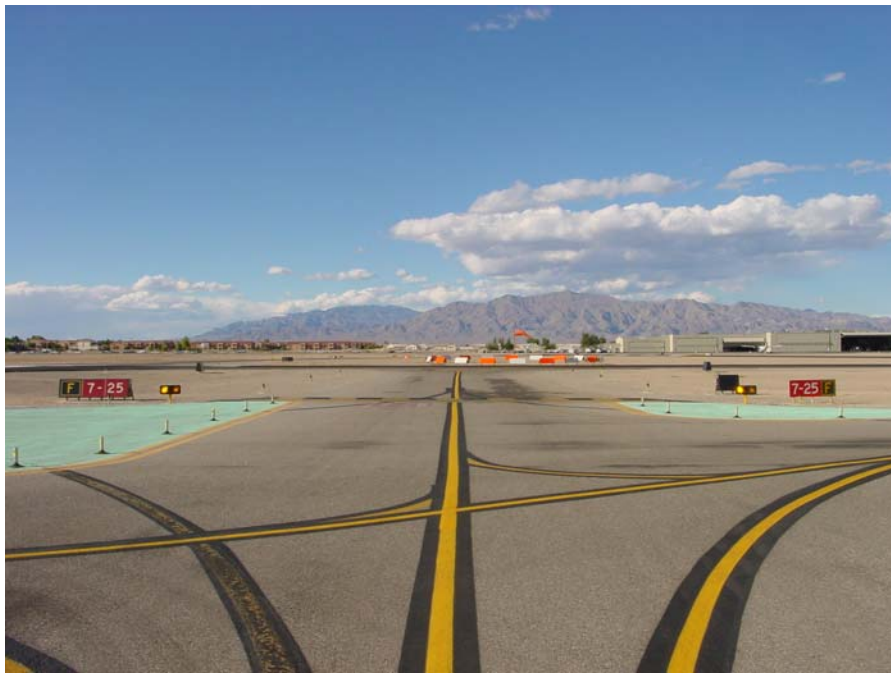
Figure A-6. Alpha 2—Runway 7-25 and Taxiway F (Southwest side)
