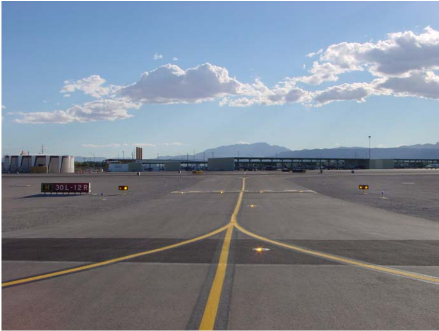
Figure A-1. Delta 1—Runway 12R-30L and Taxiway H (Northeast side)
