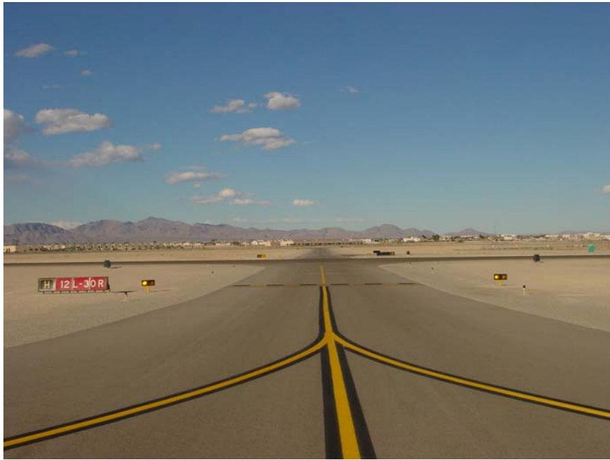
Figure A-3. Delta 3—Runway 12L-30R and Taxiway H (Southwest side)
