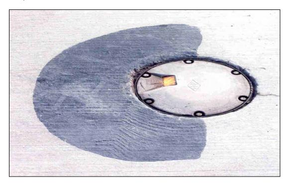
FIGURE 3. CHAMFER PAINTED BLACK IN AN EFFORT TO ABSORB AND REFLECT THE LIGHT UPWARD
