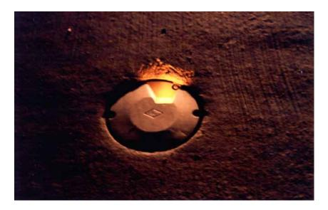
FIGURE 4. AN RGL FIXTURE WITH LIGHT REFLECTING OFF THE EDGE OF THE CONCRETE
