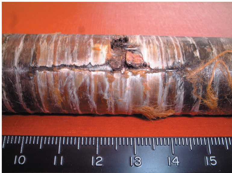
Figure 2. Layer 1 mid-plane fault illustrating short between turns.
