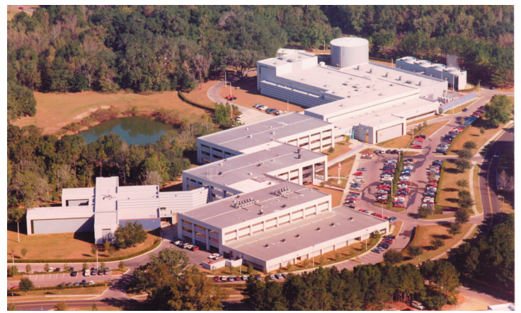
The vacant building before it became the National High Magnetic Field Facility. Two extensions were added, the NMR/ICR wing to the left, and the user facility for resistive and hybrid magnets, housing 16 magnet stations. The 26 MW cooling towers and the 4000 m 3 reservoir for chilled cooling water are at the far end.
