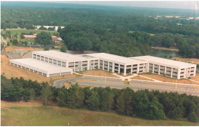
The vacant building before it became the National High Magnetic Field Facility. Two extensions were added, the NMR/ICR wing to the left, and the user facility for resistive and hybrid magnets, housing 16 magnet stations. The 26 MW cooling towers and the 4000 m 3 reservoir for chilled cooling water are at the far end.
