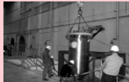
Mike Pacheco (kneeling) supervises the moving of the 60 T Long-Pulse magnet into a new pit located in the Long-Pulse Magnet Building. For safety, this building will be evacuated during 60 T Long-Pulse operations. In the background (at left) is the passage through the two-meter thick safety wall into the New Experimental Hall.
