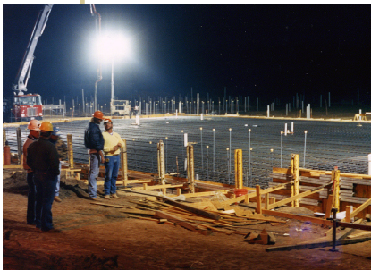
Construction of the Magnet Lab.
