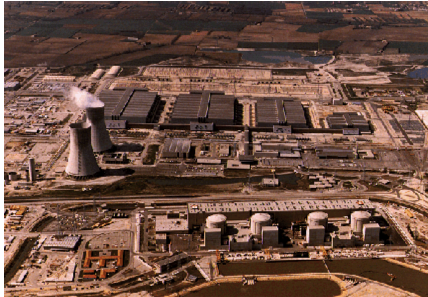
Figure C1-6. George Besse Gaseous Diffusion Enrichment Plant.
