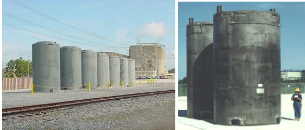
Figure E2-8. Typical dry storage casks.
