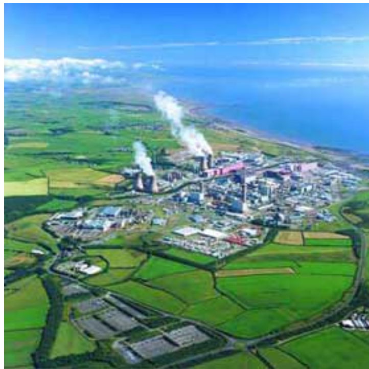
Figure F1-3. Sellafield facility, including THORP reprocessing plant (British Nuclear Fuels, plc).
