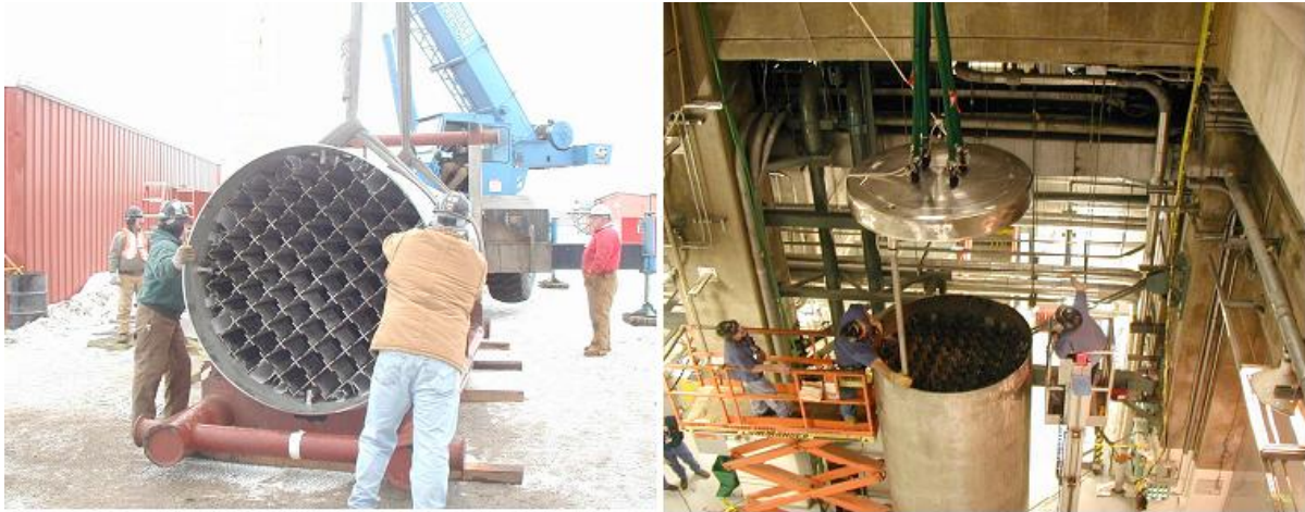
Figure E2-4. Left: Receiving the MPC at J. A. FitzPatrick Nuclear Plant. Right: Fit up of the MPC and MPC lid at J. A. FitzPatrick Nuclear Plant.
