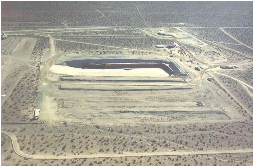
Figure J-3. Nevada Test Site low-level waste disposal facility aerial view (see Reference 1).
