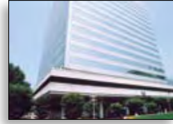
January 25 NYPA's White Plains office building receives national recognition from U.S. Green Building Council for environmental sustainability.
