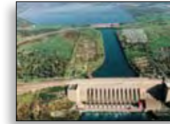
September 1 Niagara Power Project's new federal operating license takes effect.
