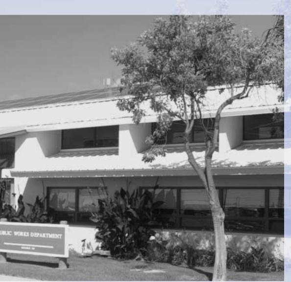
more efficient than California's 1995 Title 24 Energy Efficiency Standards. Energy efficiency was achieved through optimization of the building envelope, minimization of internal energy loads, and on-site power generation from renewable sources. The building envelope is oriented to maximize daylighting and natural ventilation, and the roof has a reflective white finish to reduce solar heat gain.
