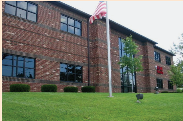
NCA's Training Center in St. Louis, Missouri, provides traditional and computer training facilities.
