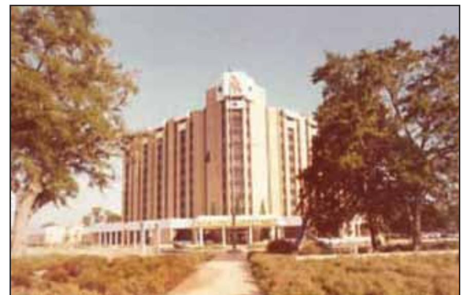
Photo of the Naval Home in Gulfport, Mississippi, in the early years.
