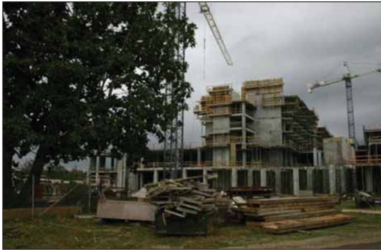
Front of building, Pavilion A.
