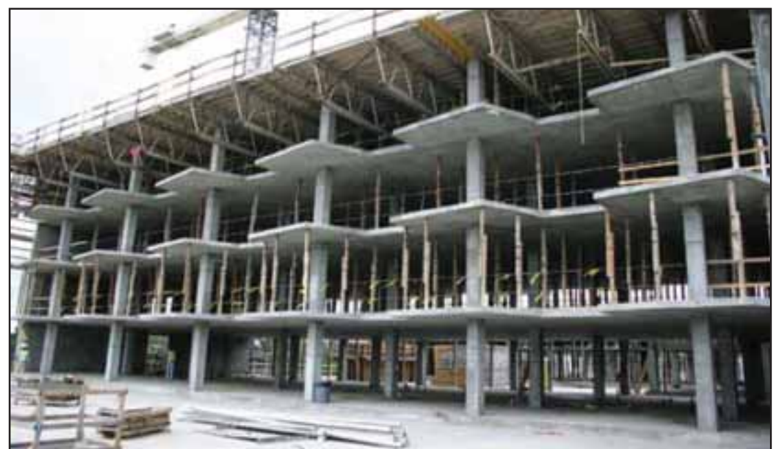
NE view of Floors 2 through 6, Pavilion A.
