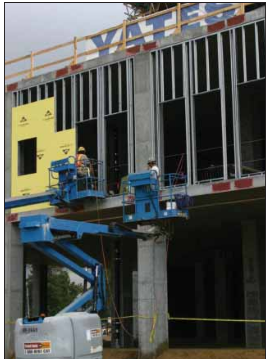
NW corner of building.
