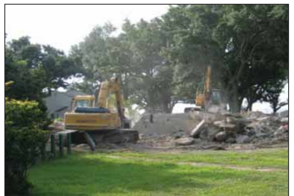
AFRH-G - demolition of the pool.
