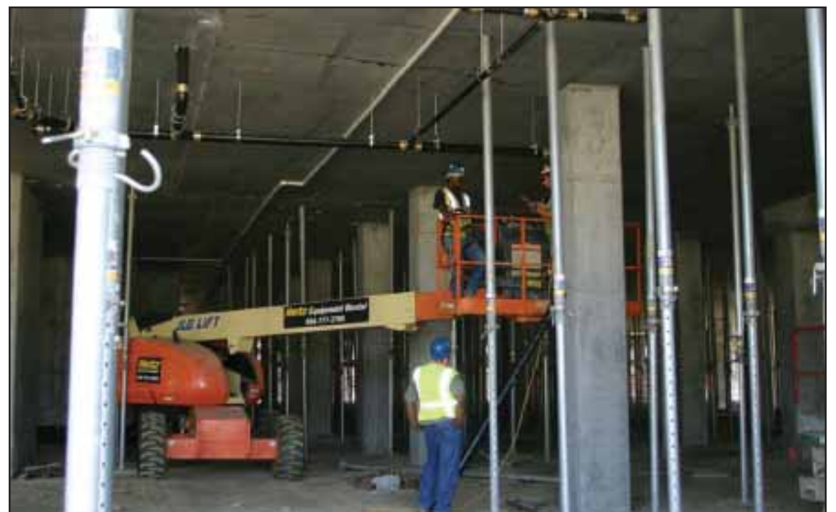
AFRH-G - view into the garage area.
