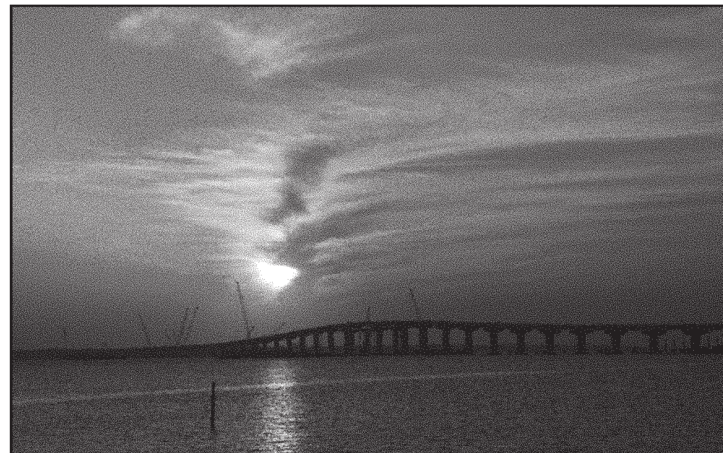
Here's a picture of the Bay St. Louis bridge from a pier in Pass Christian looking west. The bridge opened with one lane each way earlier this month.
