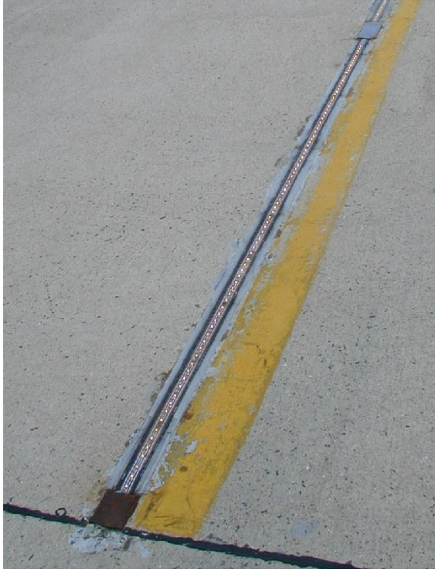
FIGURE 3. LED-STRIP SECTION PHOTOGRAPH
