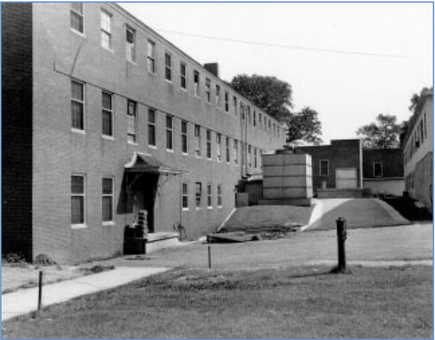
U.S. Navy Communications Annex, Building 4
