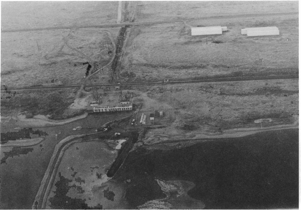
Figure 12.—Aerial view of Lorin Munn's water withdrawal site showing single, large, screened intake pipe.
