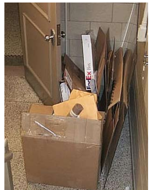
Figure 3: Storage blocking an exit pathway in a stairwell
