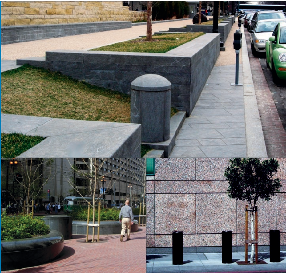
Figure 4-5: Top: Combination of low retaining walls and low bollards. Bottom, left: Combination of oversize bollard and large planters placed on very wide sidewalk. Bottom, right: Combination of tree and bollards.
