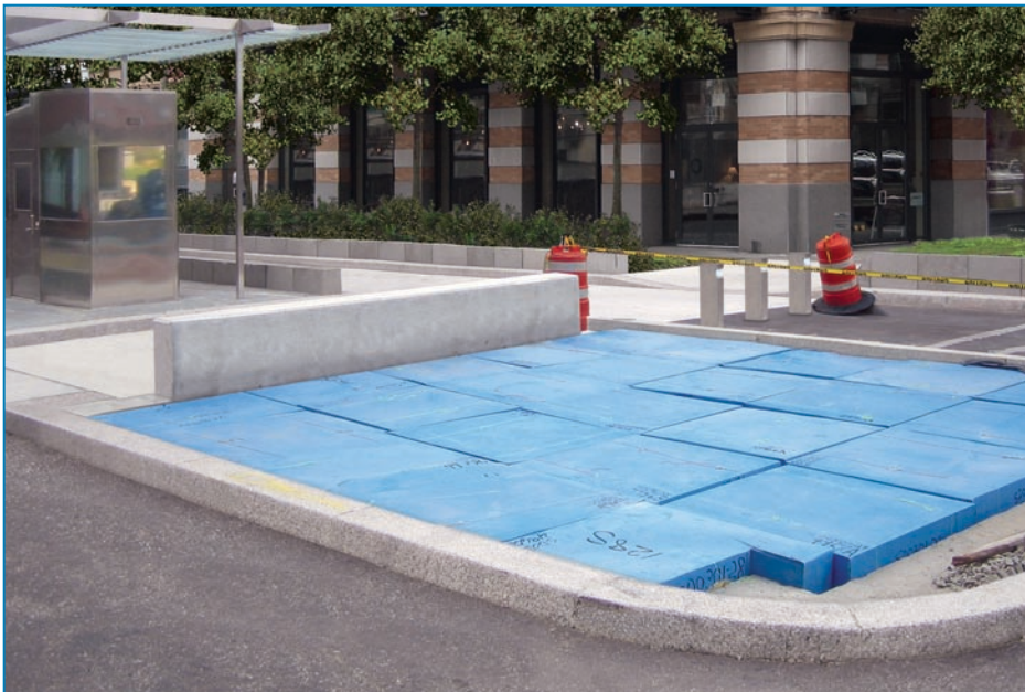
Figure 4-47: Planting cover layer creates a TigerTrap planting with a rear bench. SOURCE: ROCK 12 SECURITY ARCHITECTURE
