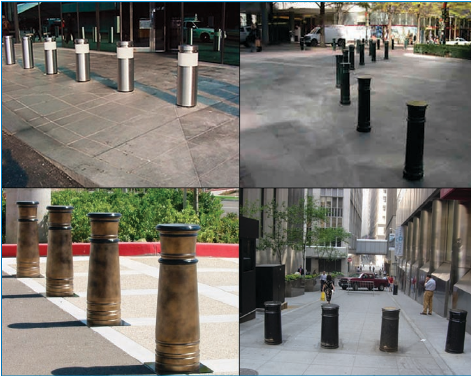
Figure 4-18: Decorative bollards with high-performance ratings.
