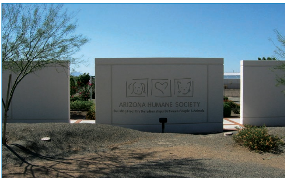
Figure 4-9: Reinforced wall barrier with artwork.
