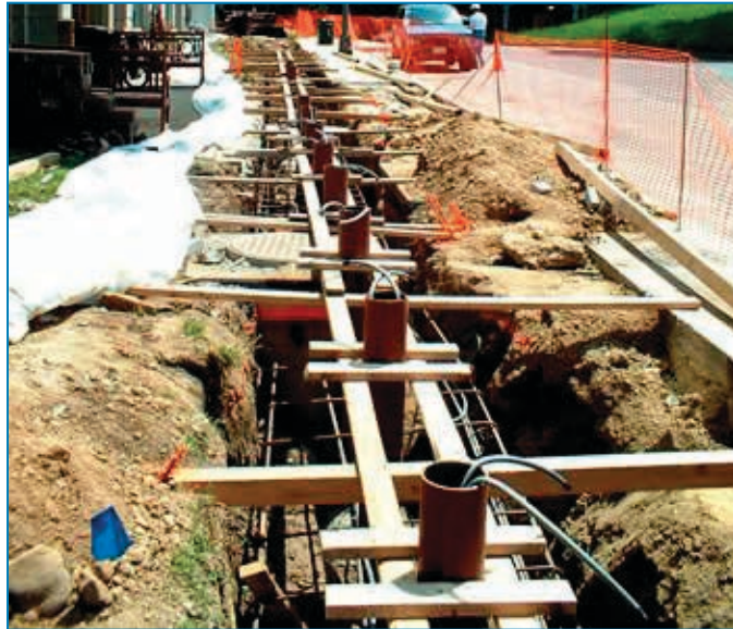
Figure 4-20: Installation of fixed bollard line. Note the depth and size of the excavation.
