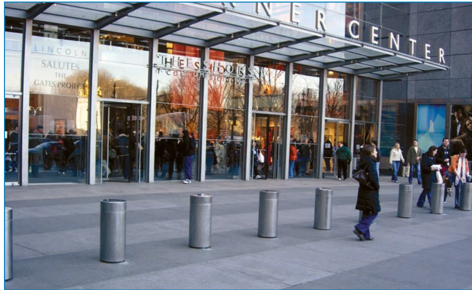
Figure 4-2: Stainless steel covers on bollards harmonize with the building entrance.
