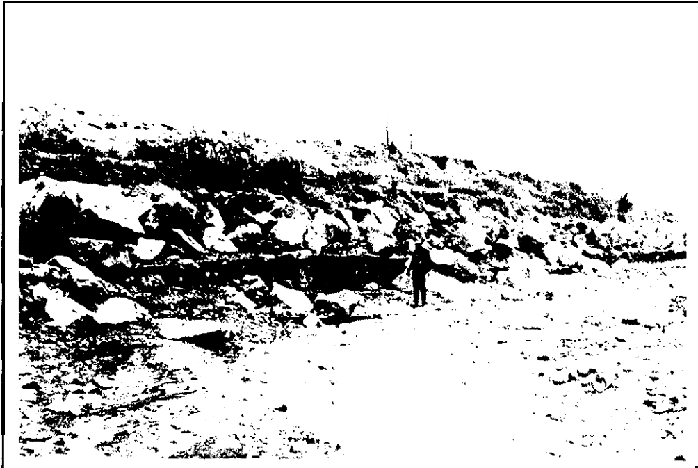
Figure 2-1 Scour Adjacent to Muscoy Groin 4 (Photo 36 - Scour depth of about three feet below the toe of grouted-stone facing.)
