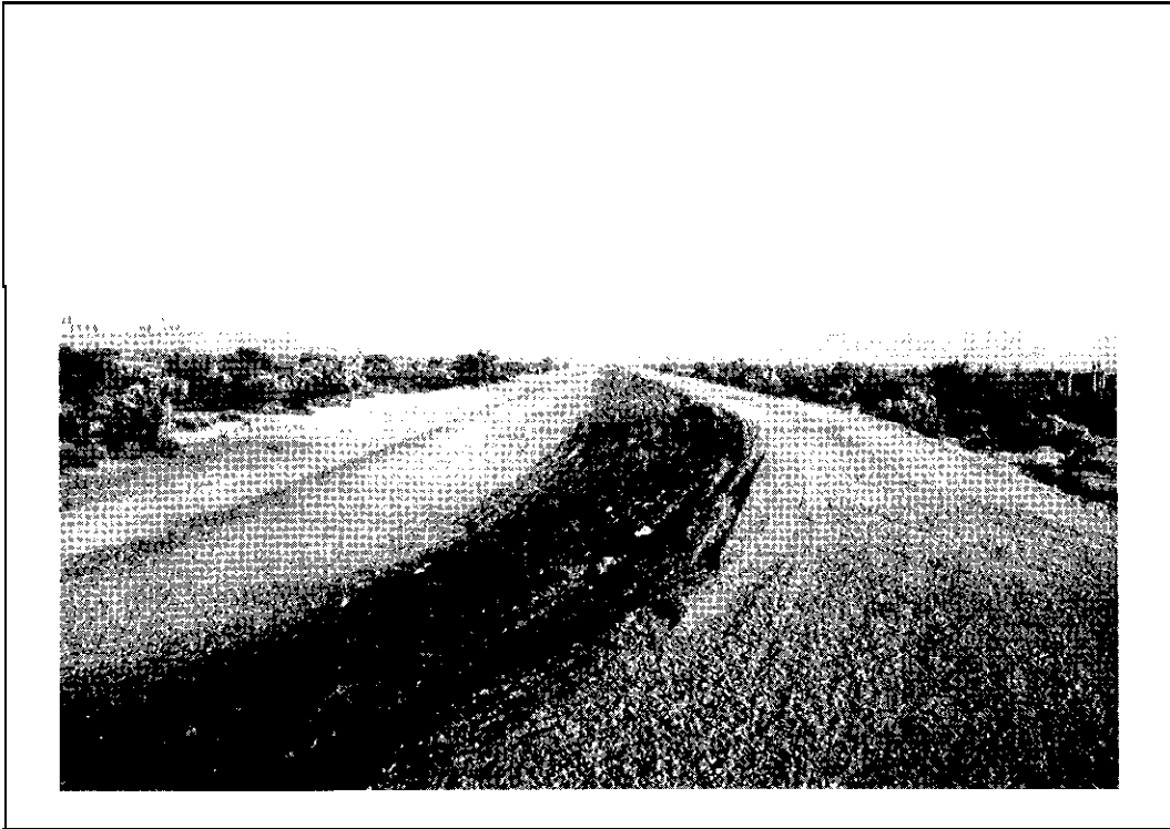
Figure 3-4 Pass Mtn. Diversion Dam, Mesa, Arizona (Flow trapped on left diverted upward in picture.)
