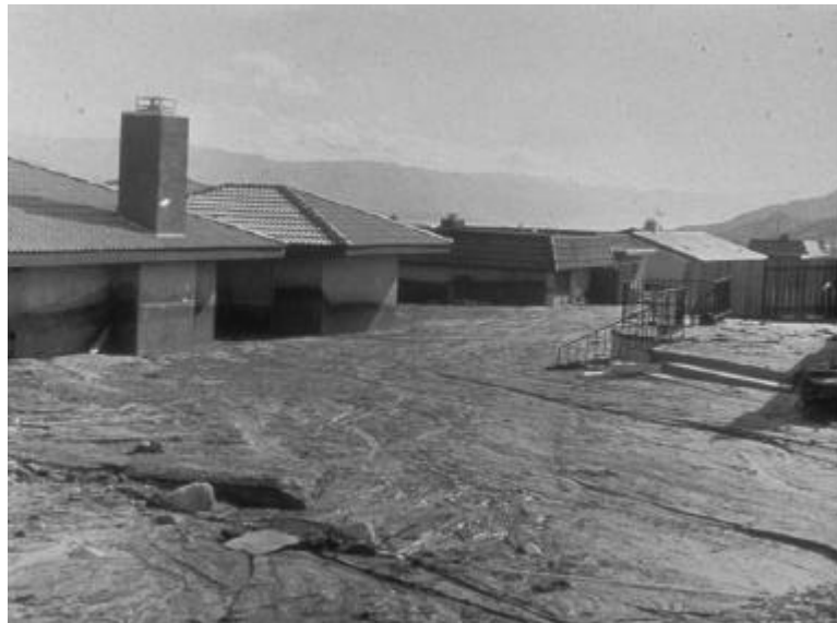
Figure 1-20. Debris flows can completely fill a house with sediment
