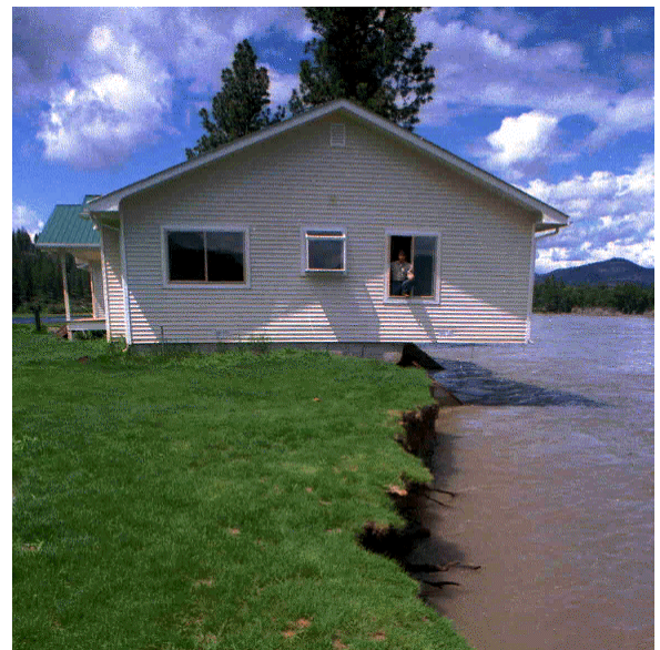
Figure 1-5. Riverine erosion can undercut structures
