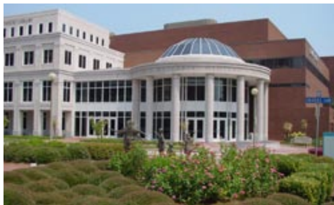
Judith Robinson, assistant dean for library and learning resources at the Edward E. Brickell Medical Services Library, teamed with architect Barry E. Moss of Tymoff & Moss to produce this addition to an existing building at the Eastern Virginia Medical School, Norfolk. Although the project was on a fast track from the start, the Robinson-Moss team still took time to include such aesthetic touches as the Jeffersonian dome.
