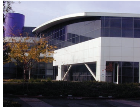
Figure 5-42: Exposed cross-bracing examples.
