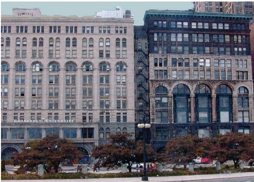
Figure 5-31 Early twentieth-century steel-frame buildings, Michigan Avenue, Chicago.
