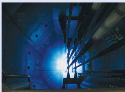
The core of the matter. The view looking down into a research reactor core in Chile shows the fuel elements and control rods hanging in a water pool.
