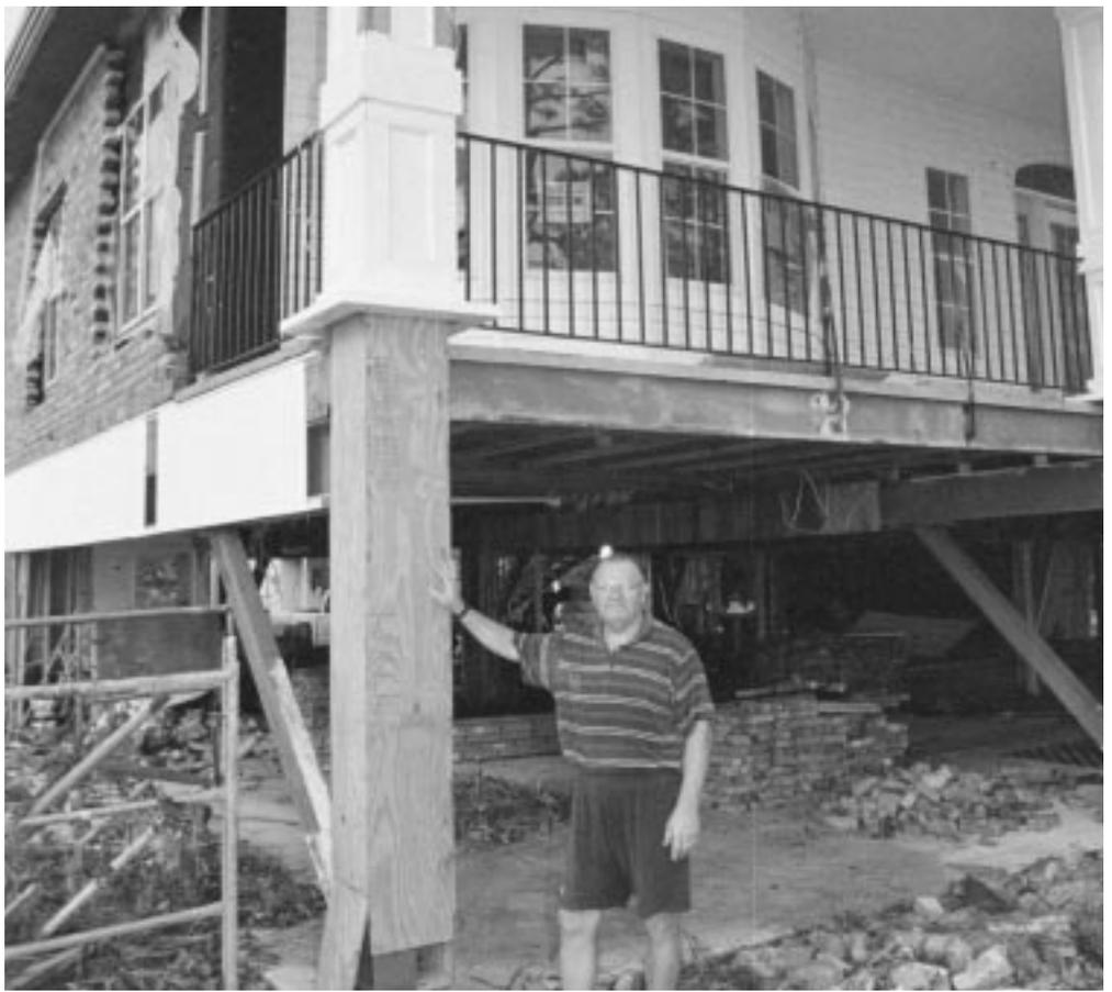
Owner stands alongside his home which was saved from Hurricane Georges by raising the structure and installing breakaway walls.
