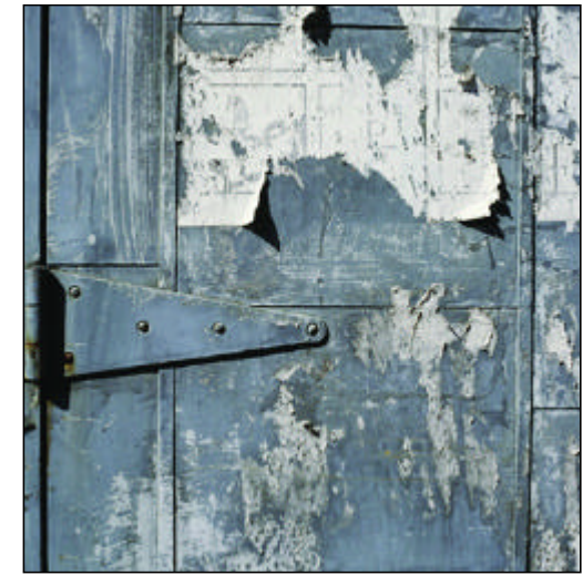
Elevated blood levels are found more often in children who live in housing built before 1950, when lead-based paint was still being used.
