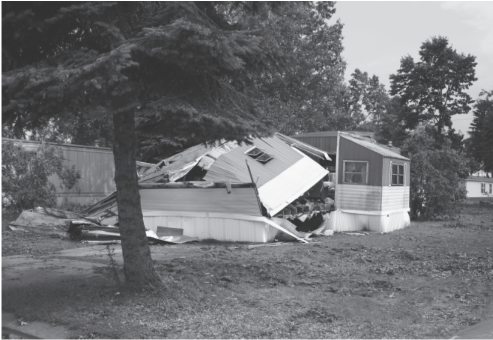
Straight Line Wind Damage—Huron County
