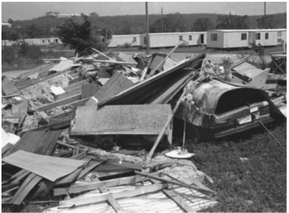
Hurricane Georges demolished a trailer in Castle Burke.
