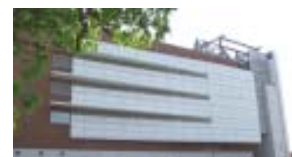
Building 11 - Power Plant
