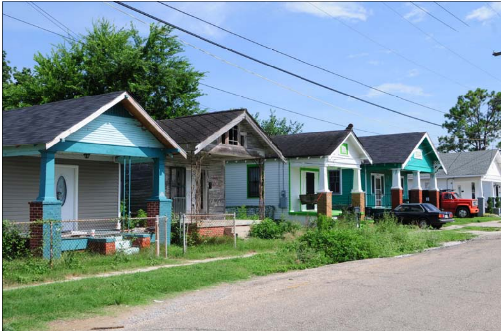
New Orleans, LA -- The resilience of the people on this block in the Lower Ninth Ward area is evident as four of the five houses have been or are being renovated. Three years after Katrina, the spirit of the people is to return "home". Barry Bahler/FEMA
