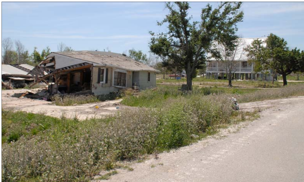
Buras, LA, -- A mitigated and non-mitigated home side by side and the resulting effects of the damage created when a Hurricane Katrina tidal surge struck. The FEMA Mitigation program is designed to minimize loss by constructing buildings that will better resist damage. Marvin Nauman/FEMA photo
