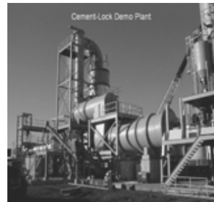
The Cement-Lock process involves heating contaminated sediment to 1400 degrees centigrade.
