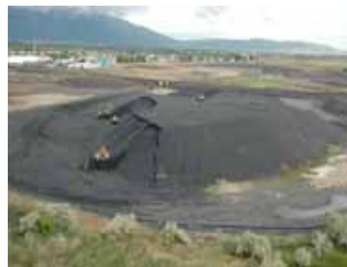
Smelter waste clean up underway.
