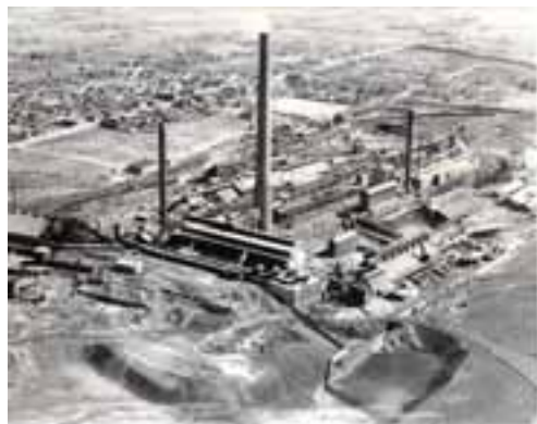
The smelter plant in the 1940s.
