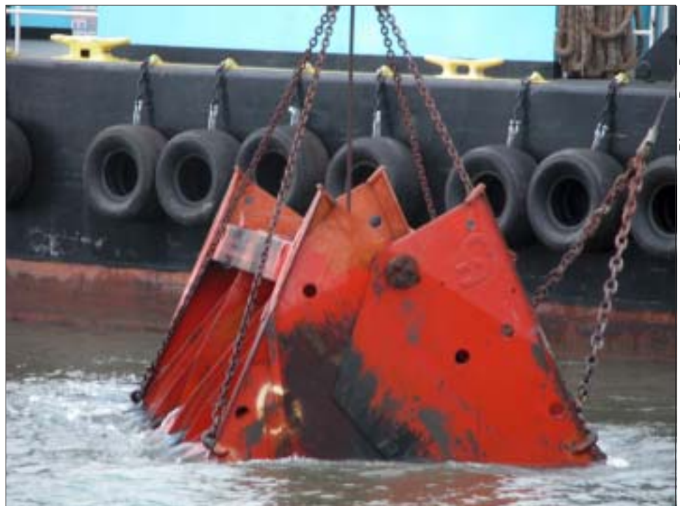
Initial dredging operations removed approximately 16,000 cubic yards of river sediment.
