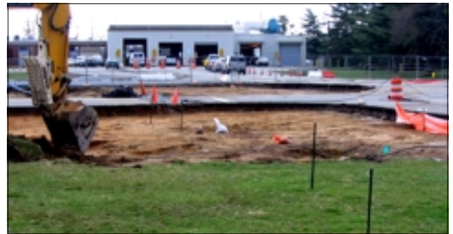
Remedial activities at the motor vehicle facility.
