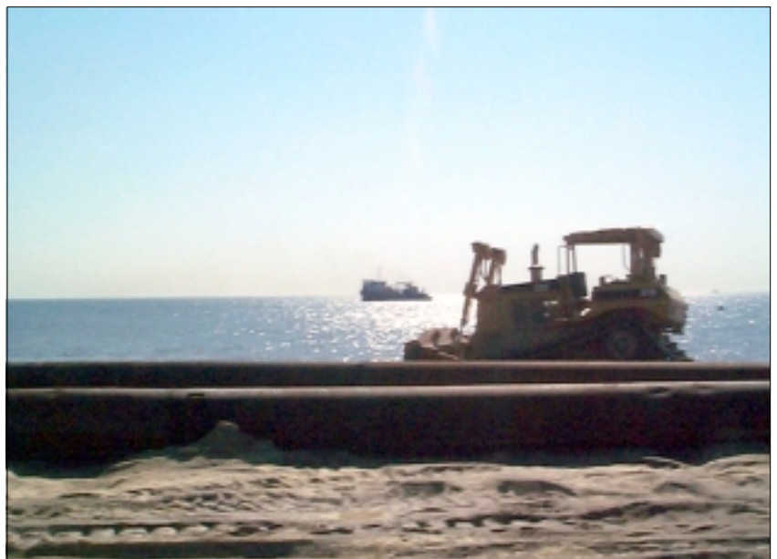
A dredge pumps sand onto the beach at Sea Bright, N.J., during a beach nourishment project.
