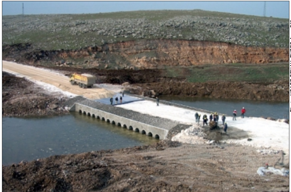
The U.S. Army Corps of Engineers provided oversight of the construction of a bridge bypass in south-central Turkey. The bypass was emplaced to accommodate the flow of heavy military equipment.
