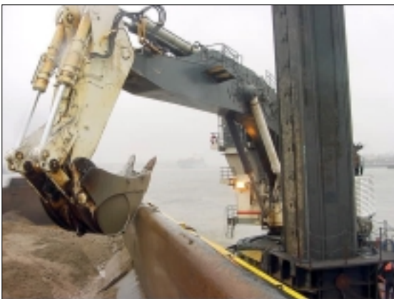
Rock glacial till material being taken from the Kill van Kull. (Photo: Larry Baier, NJ DEP)
