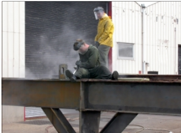
(Left) Divers use a high-pressure water blaster at 40,000 psi to refurbish a boat lift. They replaced the decking, removed rust, painted and made repairs to the structural bracing.
