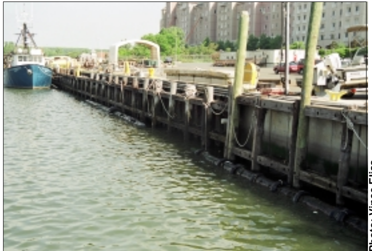
(Above) Quay wall and parking lot at Caven Point. The divers fortified the area which began to lose its fill and integrity due to years of wave action in the tidal zone.
