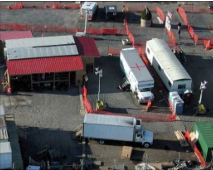
Equipment was dismantled and trailer facilities permanently closed, signalling an end to the recovery efforts at the landfill.
