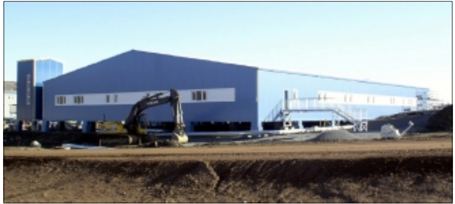
Construction of the new medical center at Thule Air Base, Greenland.
