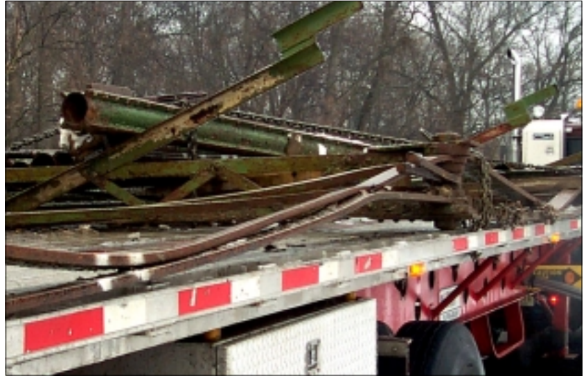
The bridge was disassembled and trucked from Oakland Borough, N.J. to Phoenixville, Pa. where it was crafted over a century ago.
