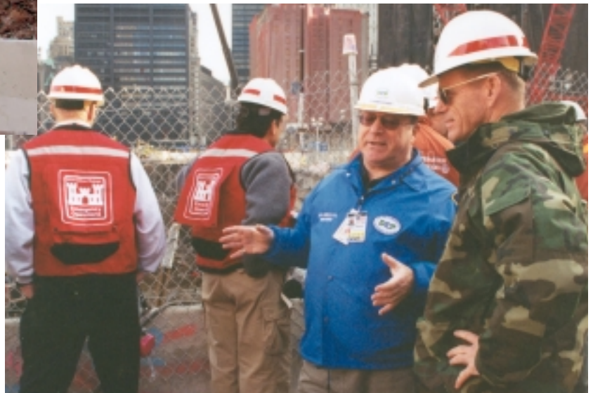
Maj. Gen. Van Winkle (right) and Joel Miele, Commissioner, N.Y.C. DEP observe the devastation and ongoing monumental task of debris removal at ground zero.
