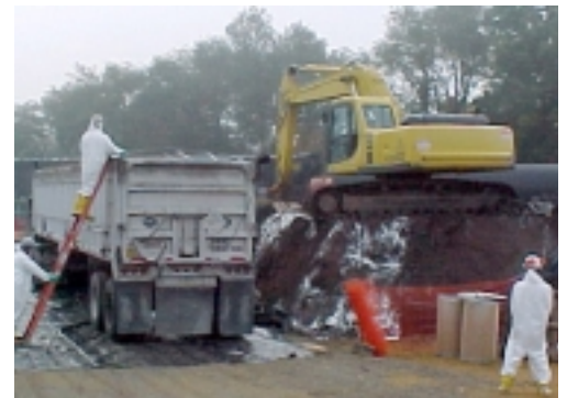
Remediation and excavation at Lagoon B.
