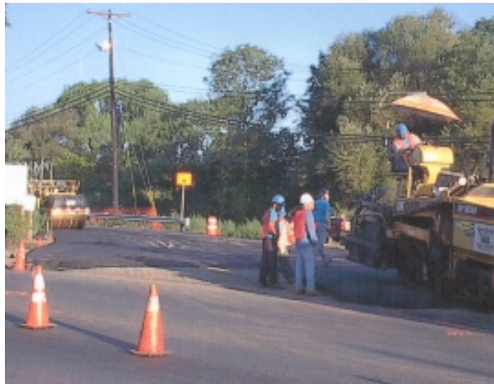
Crews pave the temporary bridge approach in Middlesex Borough.
