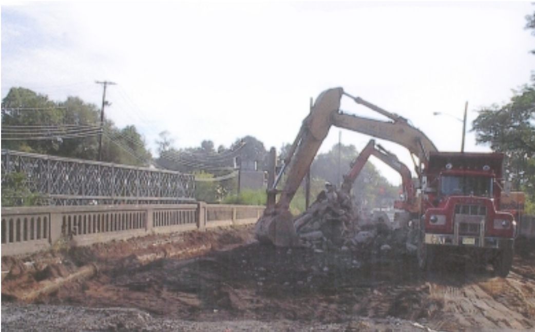
Green Brook Flood Control Project, East Main St. Bridge Demolition, Oct. 17, 2001.
