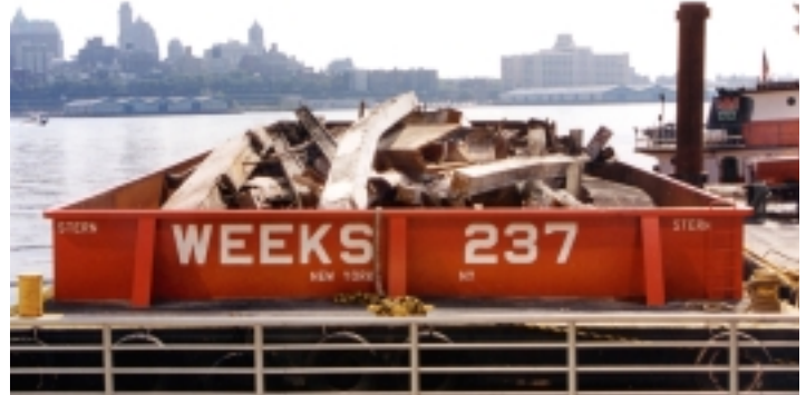
Each barge holds several thousand tons of debris.
